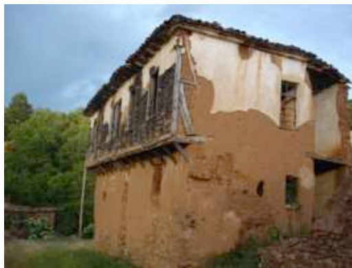
Fig. 8 -The sahnisi is deployed along the entire length of this house’s façade in Ano Kranionas village. Photo: Athanassios Balasas, Nafsika Exintaveloni, 2009
